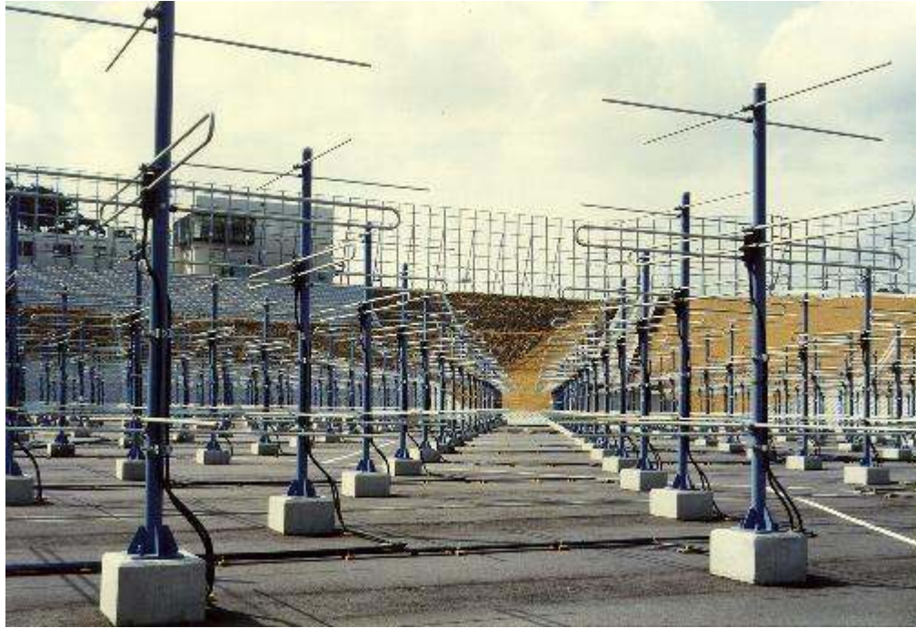
Mu Radar Yagi Antenna Elements
