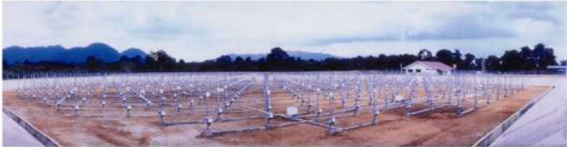
Circular array of 560 Yagi antennas (110m in diameter)
