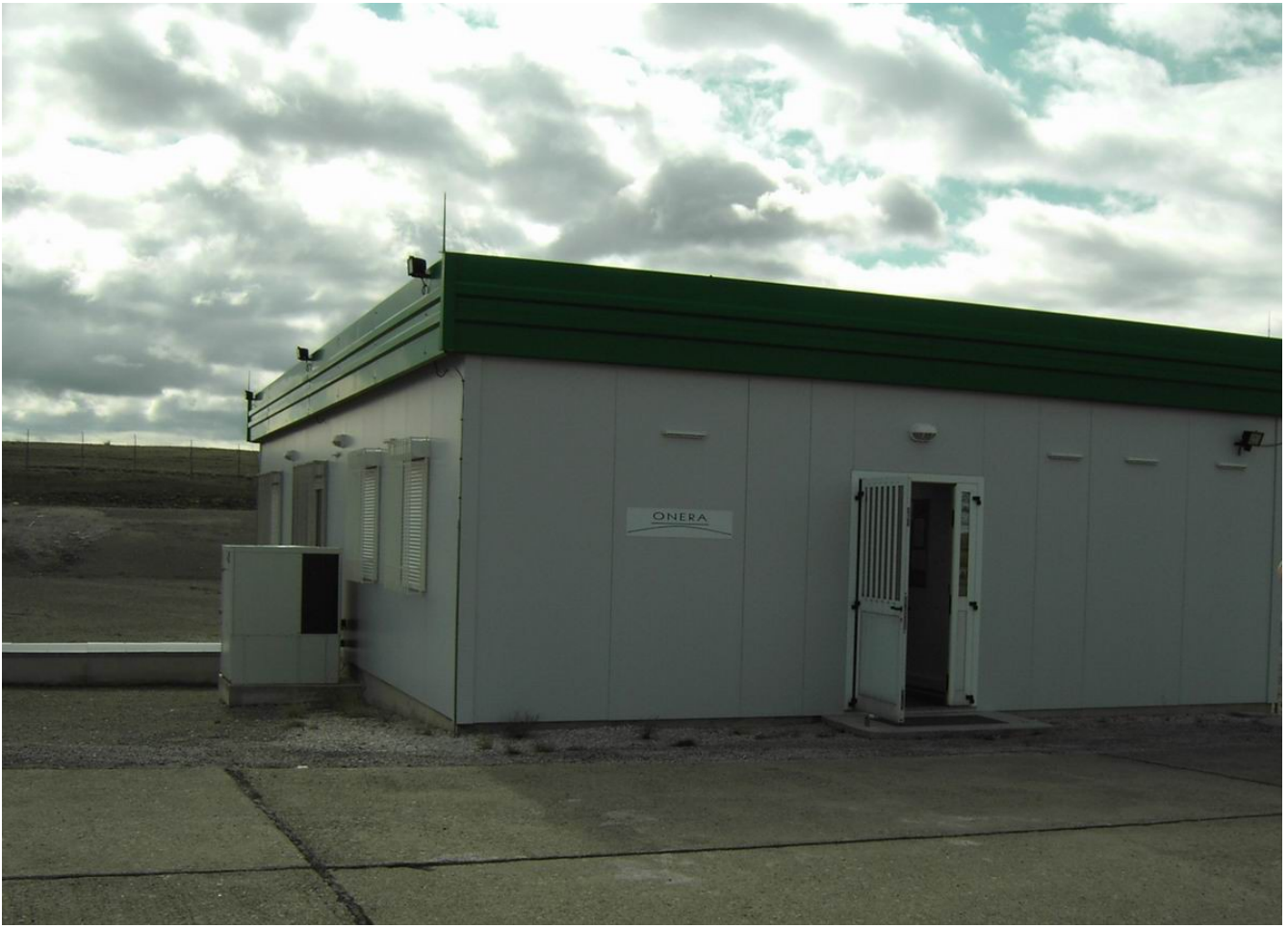
[GRAVES Receiver Building]
