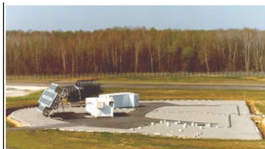
FIG 4: The GRAVES VHF transmitter station at Dijon, France.
