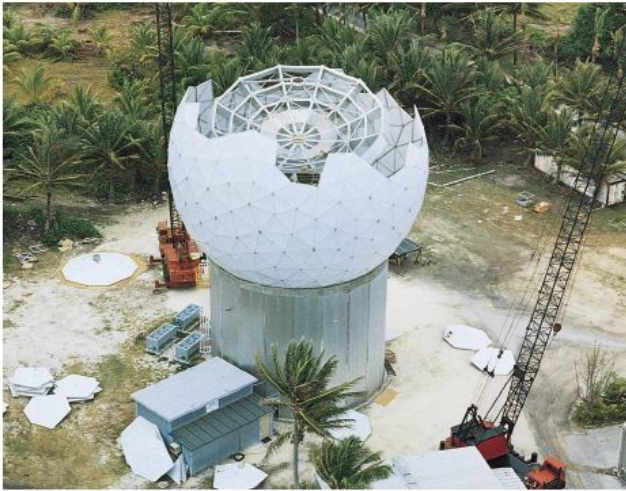
FIGURE 5. The forty-five-foot millimeter-wave (MMW) antenna and its sixty-eight-foot radome under construction on Roi-Namur Island at Kwajalein. The MMW radar was built to extend the general imaging and tracking capabilities of ALCOR and to develop millimeter-wavelength signatures of ballistic missile components.
