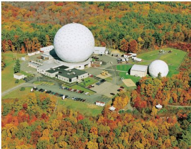
FIGURE 4. The Haystack radar site in Tyngsboro, Massachusetts. The 150-foot LRIR Haystack radome and 120-foot antenna are on the left, and the fifty-foot Haystack Auxiliary Radar (HAX) radome, forty-foot HAX antenna, and equipment building are on the right.
