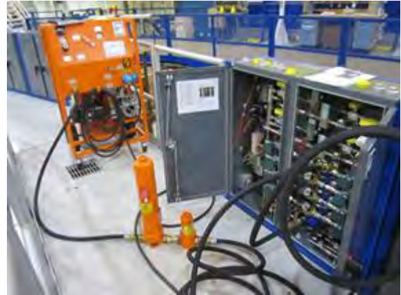
Sulfur hexafluoride reclaiming system being used on Sandia National Laboratories' Z Machine
