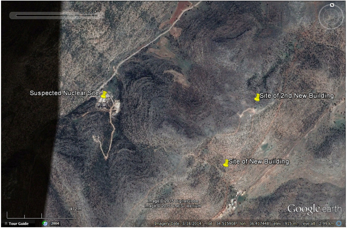
Image of 2014-03-18 showing second trail and second new building.
