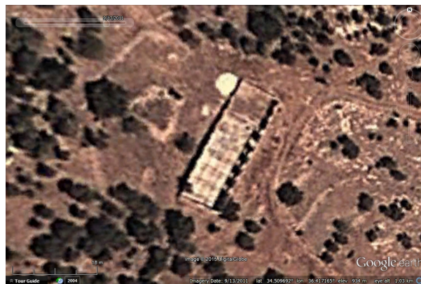
Close-up of new building, 2011-09-13
