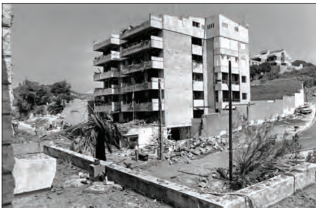
Figure 20: The Baaklini Building in East Beirut following the September 20, 1984, terrorist bombing. A suicide bomber sped into the compound and exploded in front of the U.S. Embassy Annex, injuring the U.S. Ambassador, the visiting British Ambassador, and RSO Alan Bigler. Source: © Associated Press.
