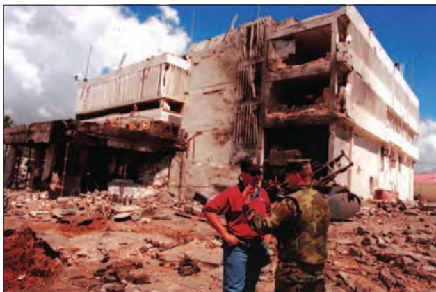
Figure 26: The damage to the U.S. Embassy in Dar es Salaam, Tanzania. The August 7, 1998, bombing occurred four minutes after the bombing in Nairobi, blowing out windows and raining debris several blocks away from the Embassy. Source: © Associated Press.
