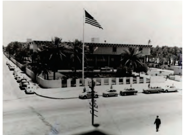
Figure 1: The U.S. Embassy in Baghdad, Iraq, circa 1975, demonstrates several challenges confronting the Security Enhancement Program (SEP). Like many embassies, the U.S. Embassy Baghdad had low perimeter walls, the walls were not solid stone or concrete, parking was allowed around the Embassy, and the building was an "open" design with large windows. The gates are also left open during the day, making the Embassy even more vulnerable. Other embassies were located in crowded city centers, making SEP upgrades more expensive and more difficult to install. Source: Department of State, Office of the Historian Files.
