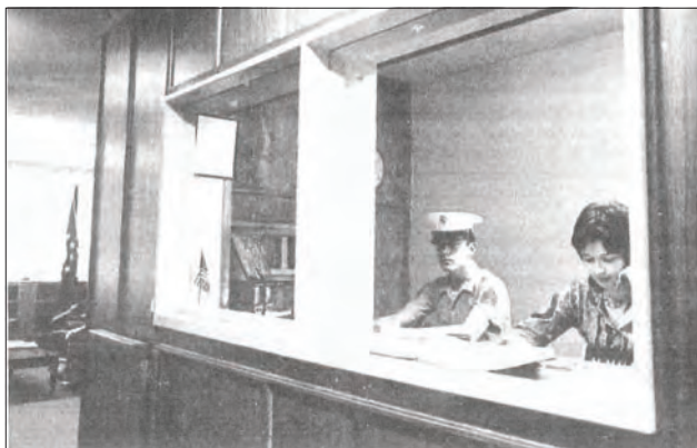
Figure 27: Marine Security Guard in a Control Booth. Under Director Victor Dikeos, SY built reinforced control booths with bulletproof glass for embassy entrances. The control booth also allowed the MSG to monitor the alarms systems and closed-circuit cameras around the embassy. Source: SY Focus.
