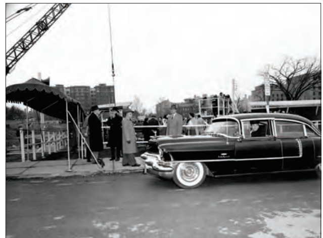
Figure 30: SY Special Agents (standing) on duty prepare for the cornerstone laying ceremony for the Department of State's new structure, now known as the Harry S Truman Building, located at 2201 C Street NW. Source: Department of State / Albert N. Abajian.
