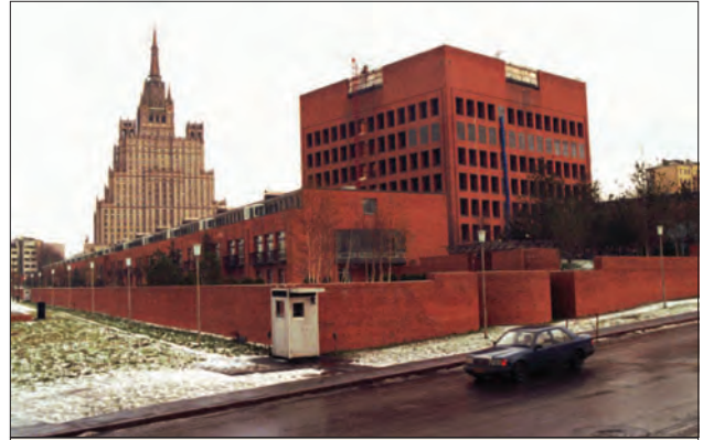
Figure 15: The New Office Building at the U.S. Embassy in Moscow. Due to the bugging system discovered in the structure of the red brick building, the United States expelled the Soviet workers, tore down the upper floors (to the base of the fifth floor), inserted shielding to prevent any new bugs, and rebuilt the upper floors. Soviet workers arranged darker colored bricks so that one could read “СССР” (Russian for USSR) in the façade of the U.S. Embassy. Source: © Associated Press.
