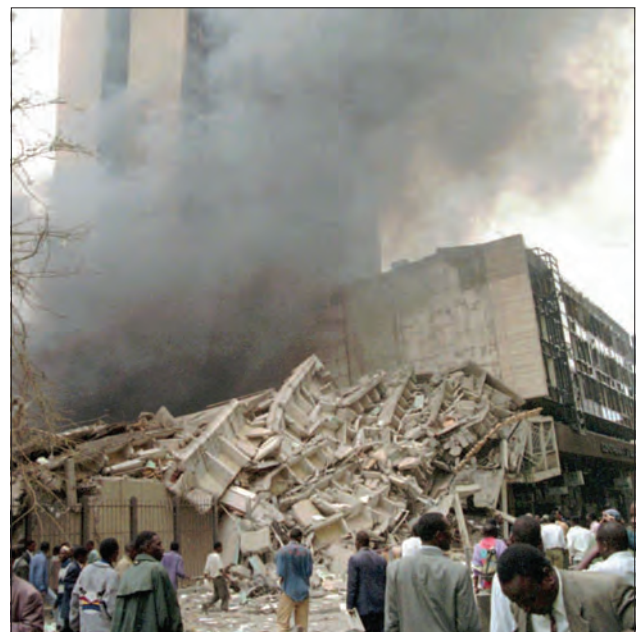
Figure 25: Damage to the U.S. Embassy in Nairobi, Kenya, shown the day after the August 7, 1998, bombing. Source: © Associated Press / Sayyid Azim.
