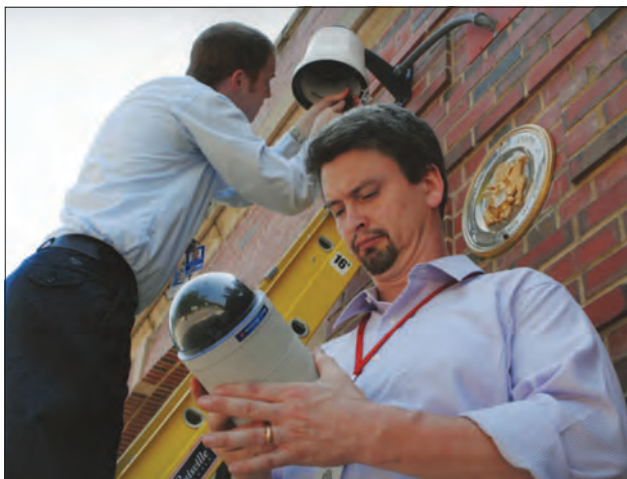
Figure 5: A DS Security Technical Specialist (foreground) inspects a surveillance camera while a DS Security Engineering Officer works on the mounting hardware at a United States diplomatic facility. Although the Cold War had ended, threats to U.S. diplomacy, such as espionage, terrorism, and crime, continued. Moreover, the United States needed to establish embassies in the newly independent states of the former Soviet Union. As a result, DS faced many challenges in ensuring the technical security of U.S. diplomatic posts during the 1990s. Source: Bureau of Diplomatic Security Files.
